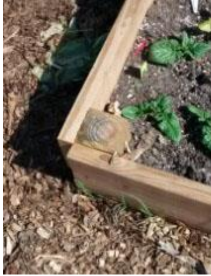
Garden frames are held together with 4x4 using galvanized screws
