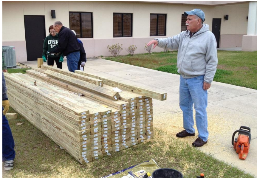
Pressure treated lumber delivered on site for the garden plot frames
